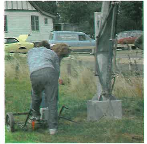
Stages in the erection of a hinged aluminium column.
