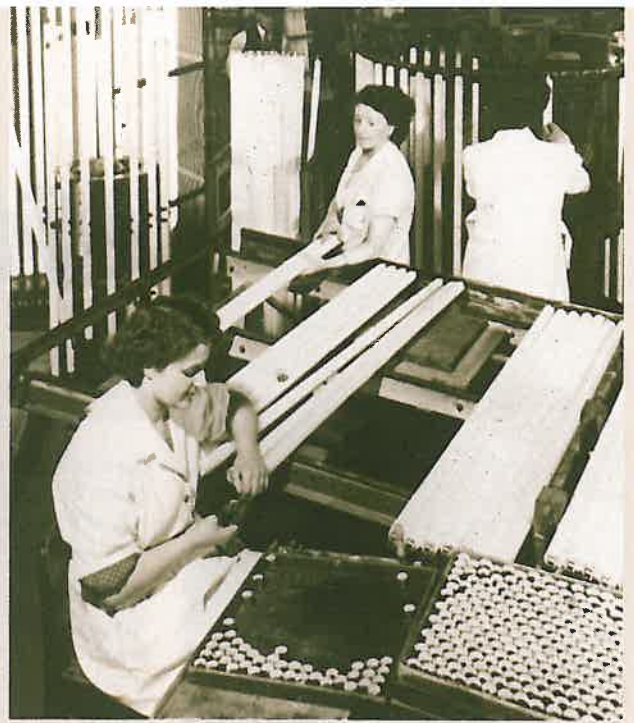
Blowing the glass tubing for fluorescent lamps was still a craft operation in the forties. The lamps themselves were assembled by hand. The picture shows capping and ageing lamps.
