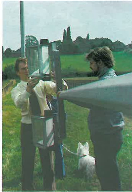
Stages in the erection of a hinged aluminium column.
