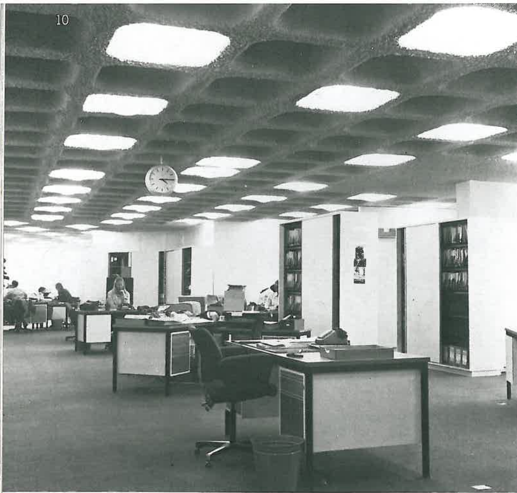
The specially designed MBF luminaires in the coffered ceiling at the Metal Box offices at Reading are located to provide the maximum illuminance at work stations.
